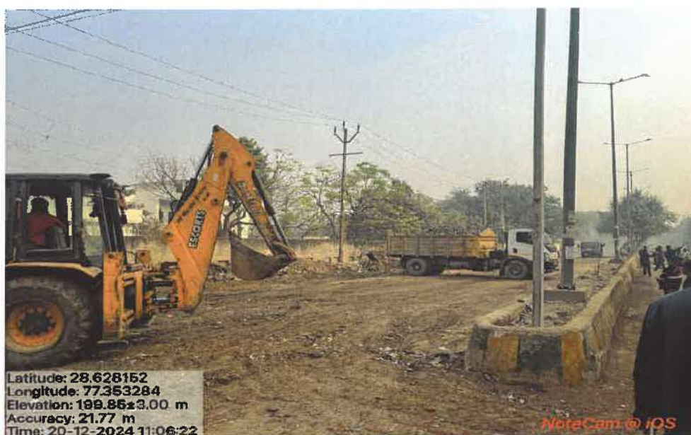
Figure 1: Site Photograph of Mixed Waste on Roads.
